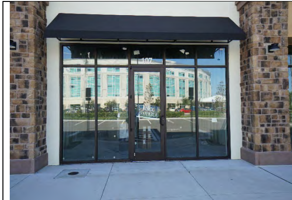
General view of exterior unit #107
