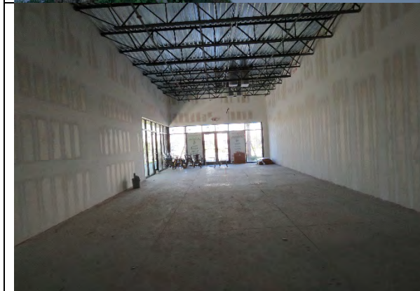
General view of interior unit # 108
